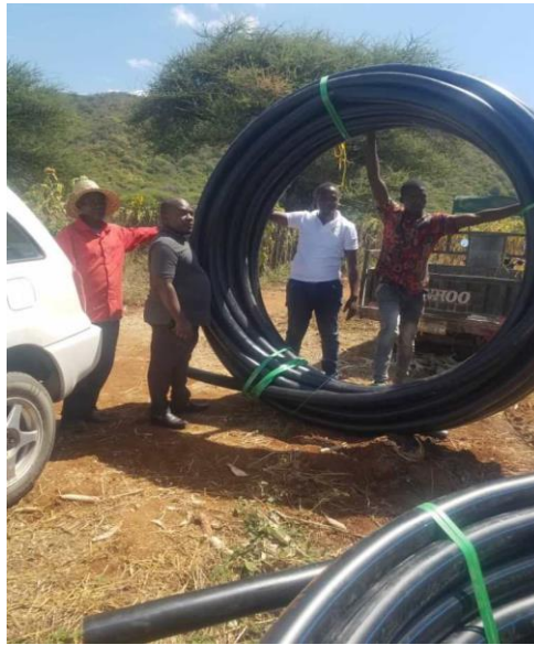
The pipes to be laid out in trenches
